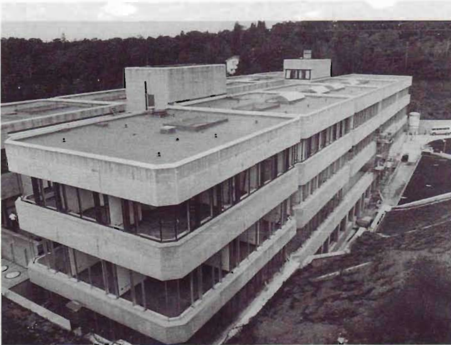
The New Building, adjoining the existing Main Building and equal to it in size. It will be occupied in early 1990.
