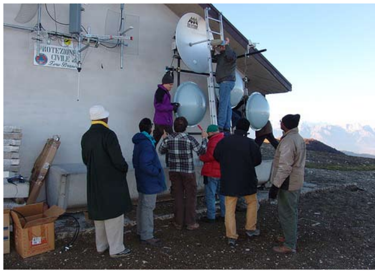
Setup and alignment of antennas in top of Mount Cesen (1500 m), Italy, by the Task Force international team (Courtesy of C. Fonda)
